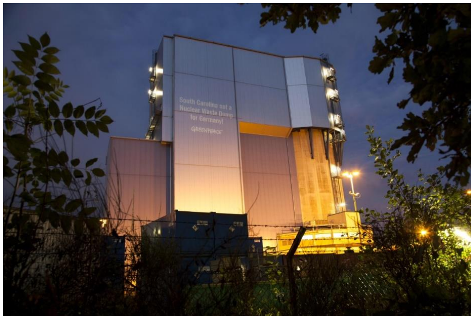
AVR reactor at the Jülicher Research Center in 2014, before its dismantlement. The reactor was subsequently removed and placed in a special storage facility on site. The words projected onto the reactor building by Greenpeace read "South Carolina not a Nuclear Waste Dump for Germany."
